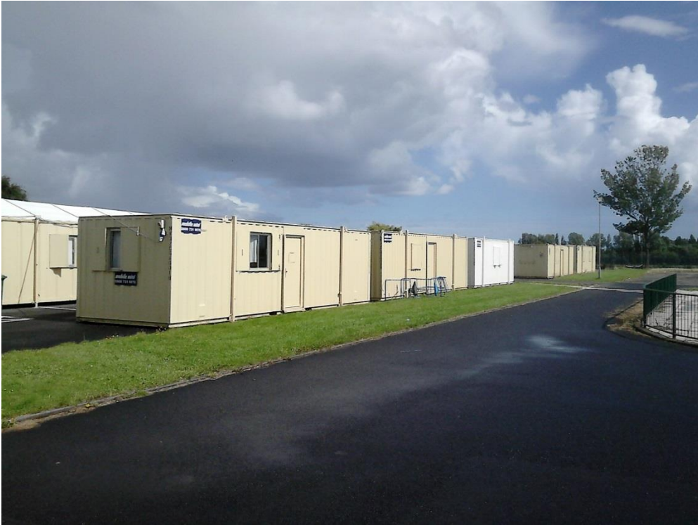
External Accommodation (Rear of Sports Block)
