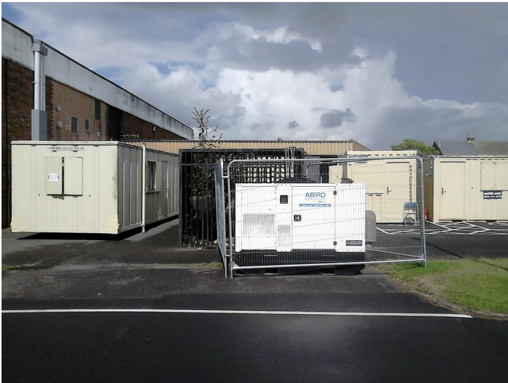
External Accommodation (Rear of Sports Block)
