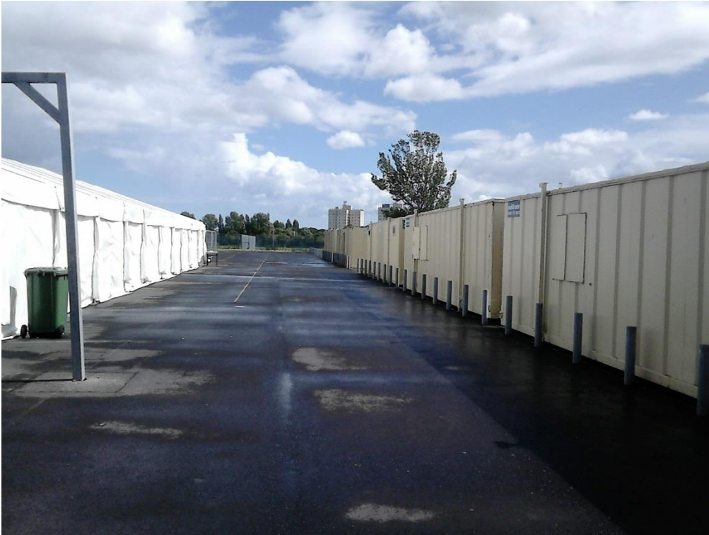
External Accommodation (Rear of Sports Block)
